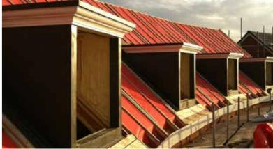
Fully insulated roof cassettes, manufactured in our controlled factory environment, achieving required U-values.
